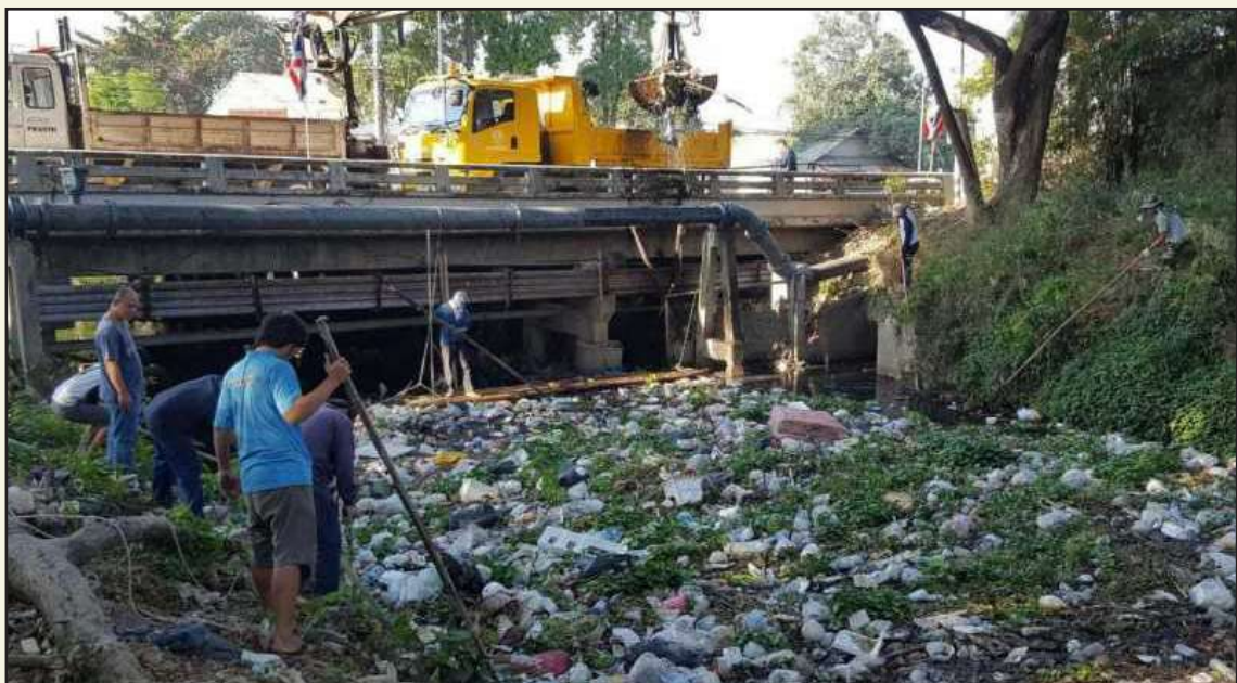
The problem of garbage blocking the Mae Kha canal, making floods more likely to occur
